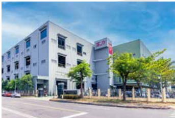
Kaohsiung Taiwan Plant
