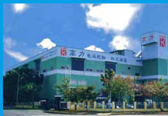
Kaohsiung Taiwan Plant
