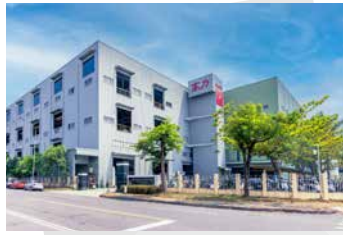
Kaohsiung Taiwan Plant
