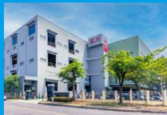
Kaohsiung Taiwan Plant
